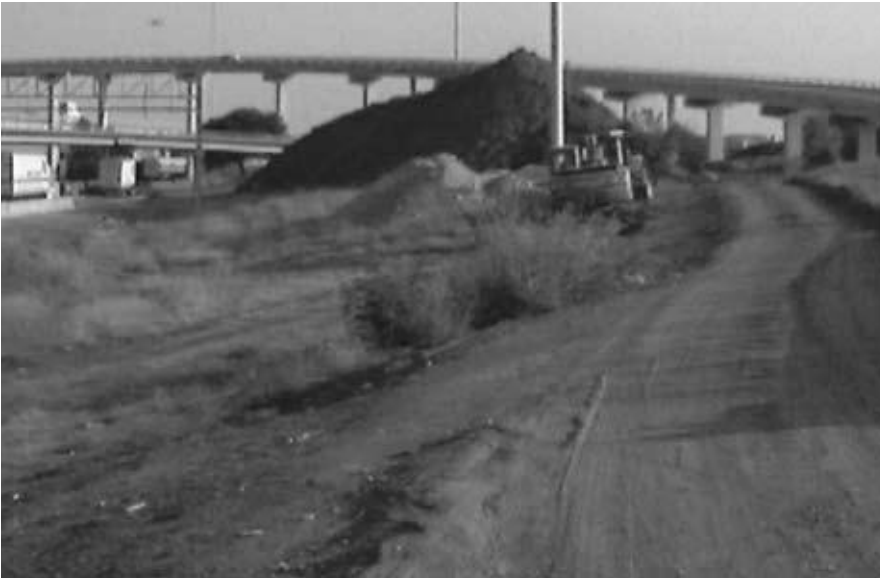
Soil tests at the construction site found that some of the soil was contaminated with metals and could not be used. Excavated soils had to be stockpiled until a determination allowed the soil to be properly disposed or reused on the project.
