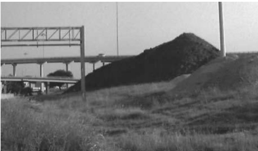
It required 1,500 soil samples to determine what soils could be recycled. The XRF equipment efficiently allowed the contaminated soil to be identified and stockpiled for proper disposal.
